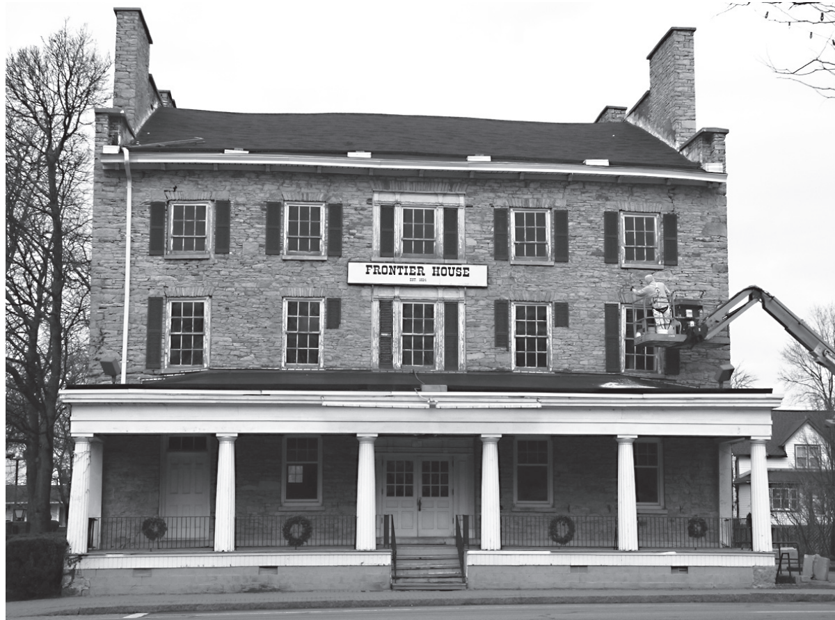
Mortar work began in December on the Frontier House.
